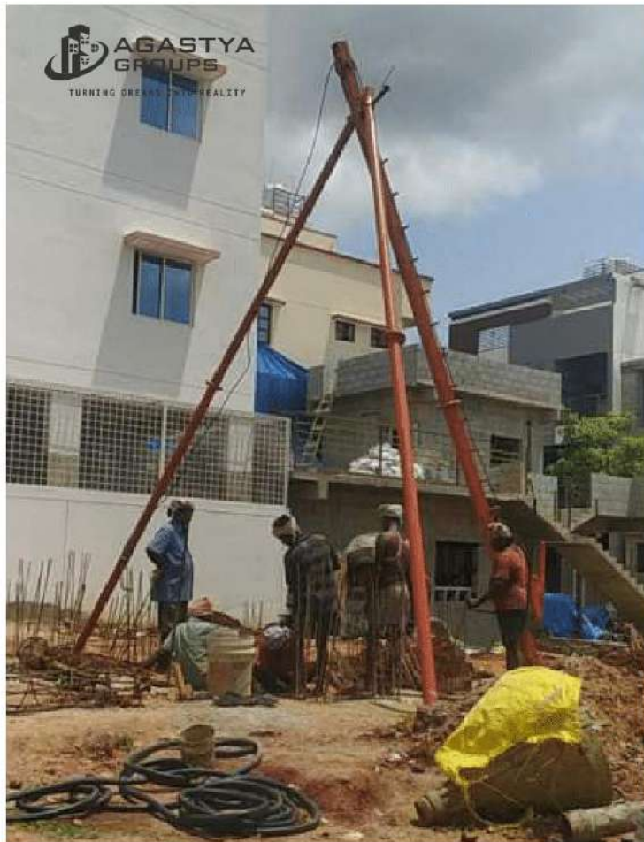
Pile footing at Mr. Swamy's project
